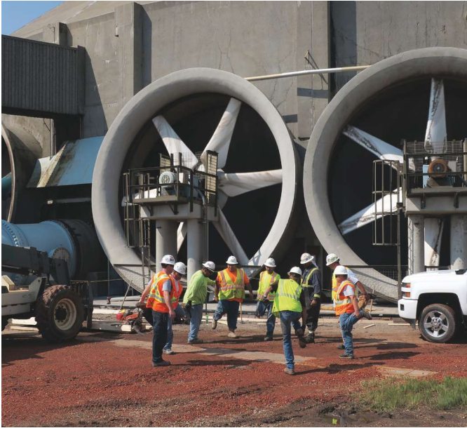
Fig. 3: Workers catch up and share stories during stretch and flex sessions at the Antelope Valley Station in North Dakota
