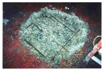
Work consisted of removing the existing failed concrete coating along with all contaminated concrete. All concrete repairs were completed with a fast setting engineered repair mortar so as to allow the installation of the coating system without the usual curing time of 28 days as with standard concrete repairs. Once the concrete repair had been completed a Ceilcote 505 fiberglass reinforced epoxy coating system was installed.
