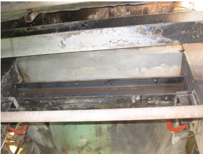
Structural Repairs Prior to Grouting
