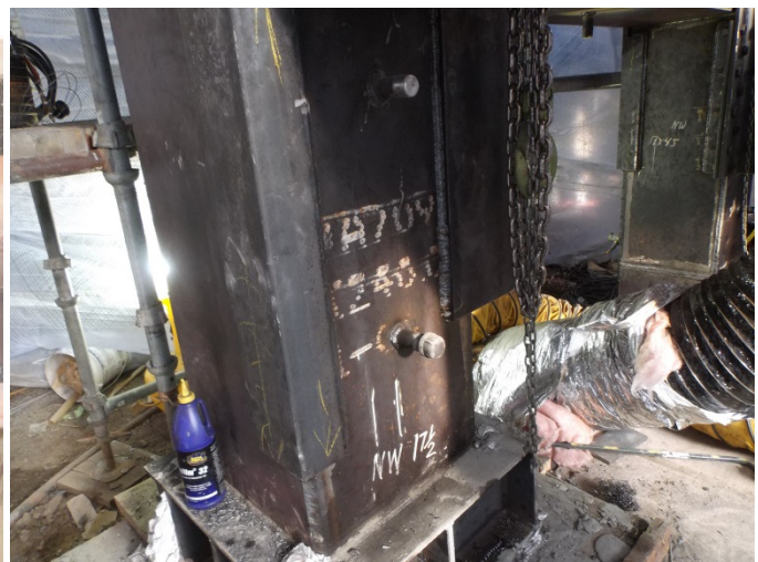
View of the Steel Encasement
